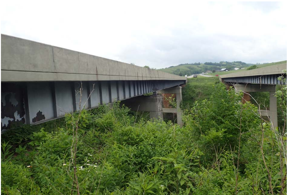
View from the north end of abutment 4.
