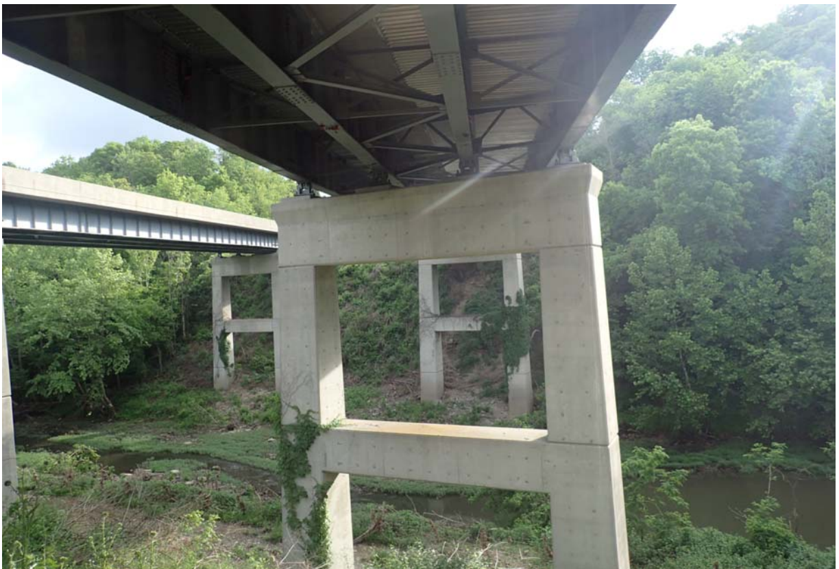
Typical view of span 1 and pier 2.
