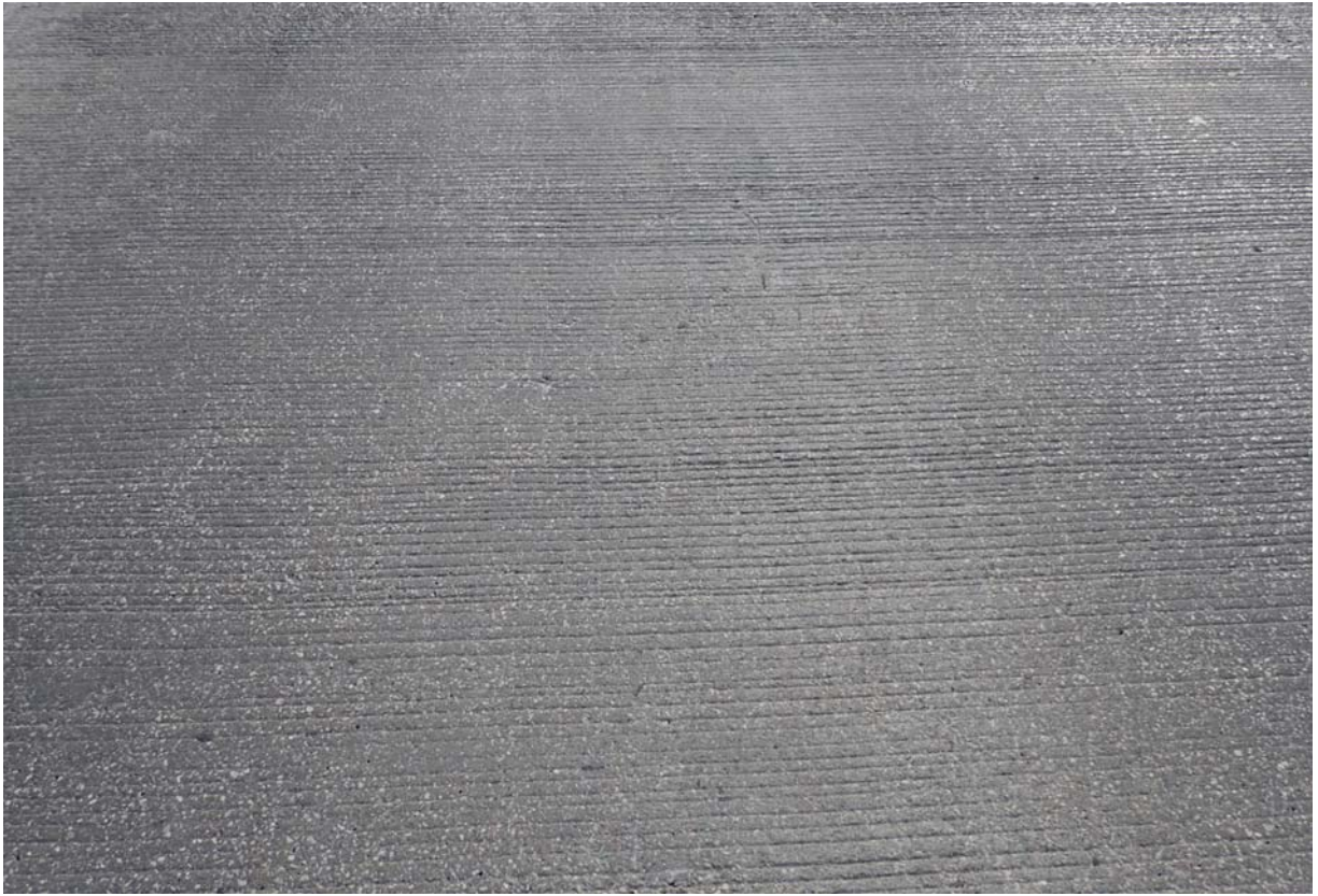
Typical view of the wearing surface.
