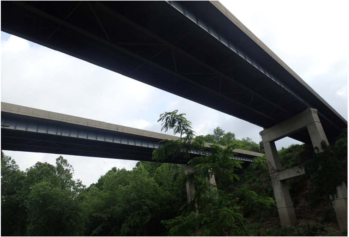
Typical view of span 2 and pier 3.
